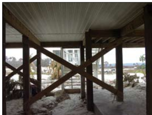
Figure 2. An open foundation.
