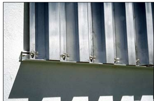
Figure 4. This metal shutter has top and bottom tracks that are permanently anchored to the wall (FEMA 577).
